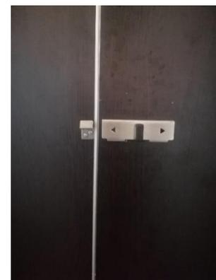
4.6.1.4.8 12 mm thk waterproof compact laminated board urinal partition including 0.5 mm stainless steel angle bracket with complete accessories. Approved type and quality.
